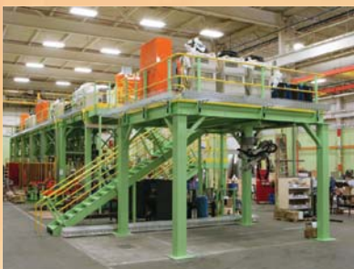
Manufacturing Mezzanine with Gantry Robot
