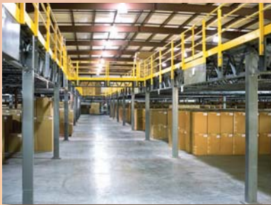
Warehouse Mezzanine with Walkway Bridge
