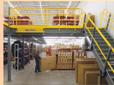
Auto Dealership Mezzanine with Slide Gate
