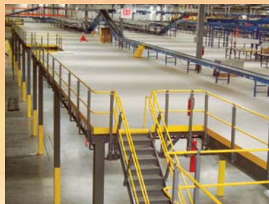
Distribution Center Mezzanine with Resin Board Floor System
