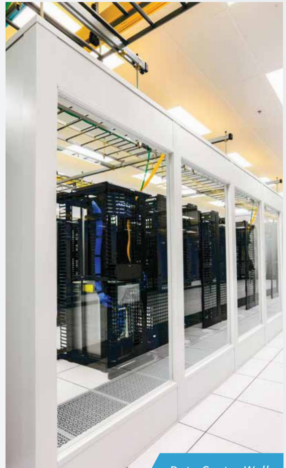
Data Center Walls
