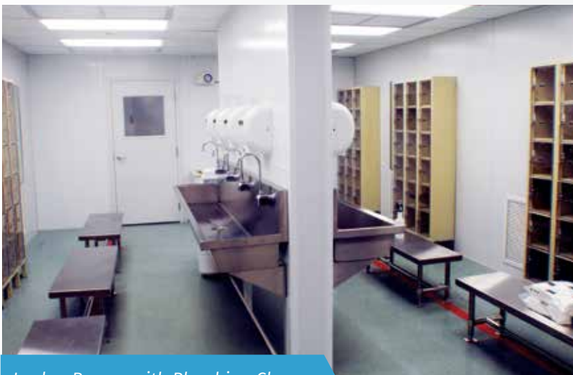
Locker Rooms with Plumbing Chase
