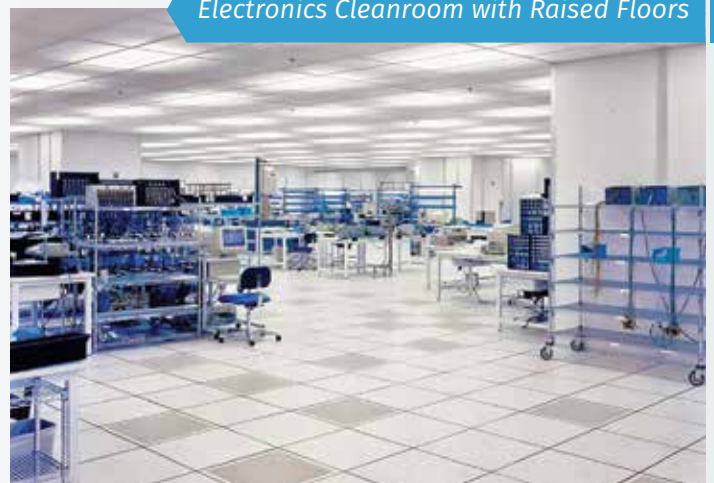
Electronics Cleanroom with Raised Floors
