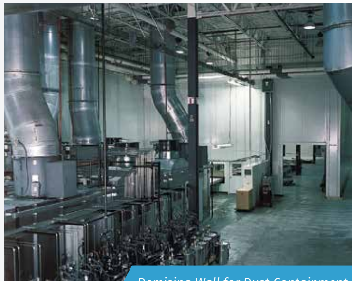
Demising Wall for Dust Containment
